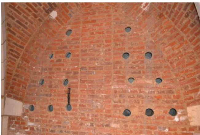
Figure 1 – Acoustical pots in the West wall of the phonocamptic cave at Noyon
