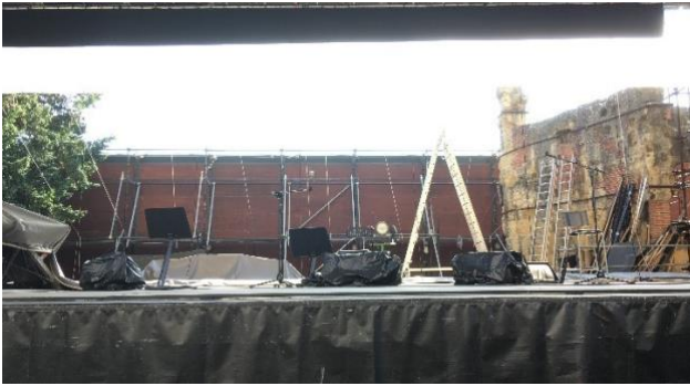
Figure 1 – View of a temporary acoustic barrier mounted behind the stage.
