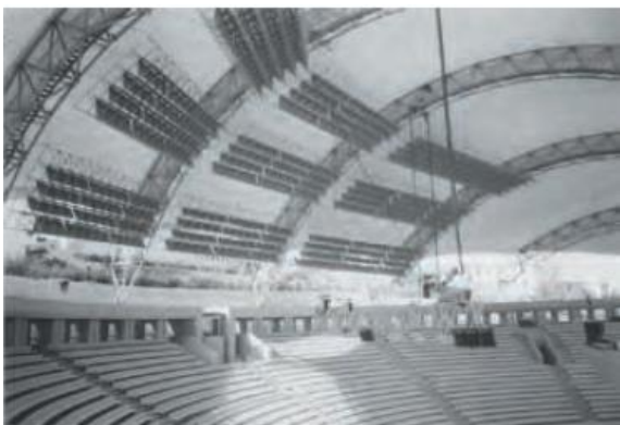
Figure 9 – Interior view showing the sound absorptive panels at the rear zone of the amphitheatre
